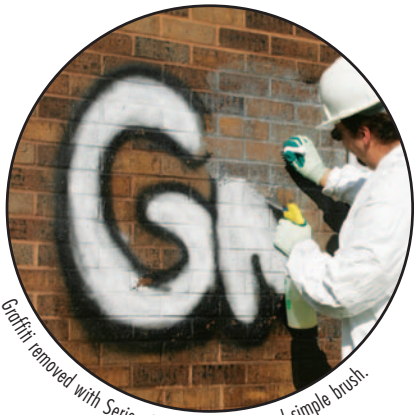
Building tagged with graffiti.
