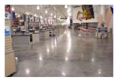
specifically sealants and adhesives, such as those used on carpet, carpet pads, rubber floors, VCT, and ceramic tile. The Ashford Formula dispenses with all of these floor coverings, since it allows exposed concrete floors to be used as the finished working surface.
