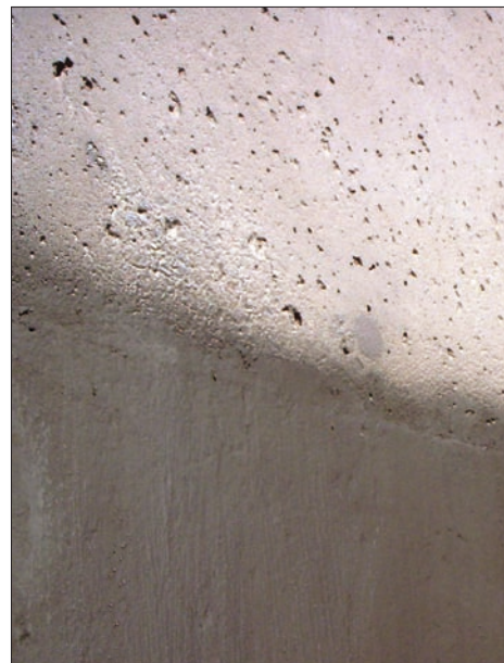
Typical cast-in-place concrete wall containing exposed bugholes (upper half of photo) and application of a greenish, epoxy-modified cementitious resurfacer (lower half).
