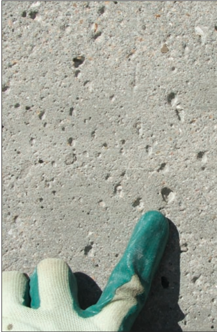
Cast-in-place concrete after SSPC-SP13/NACE 6 surface preparation to expose bugholes and create an anchor profile according to ICRI-CSP5.
