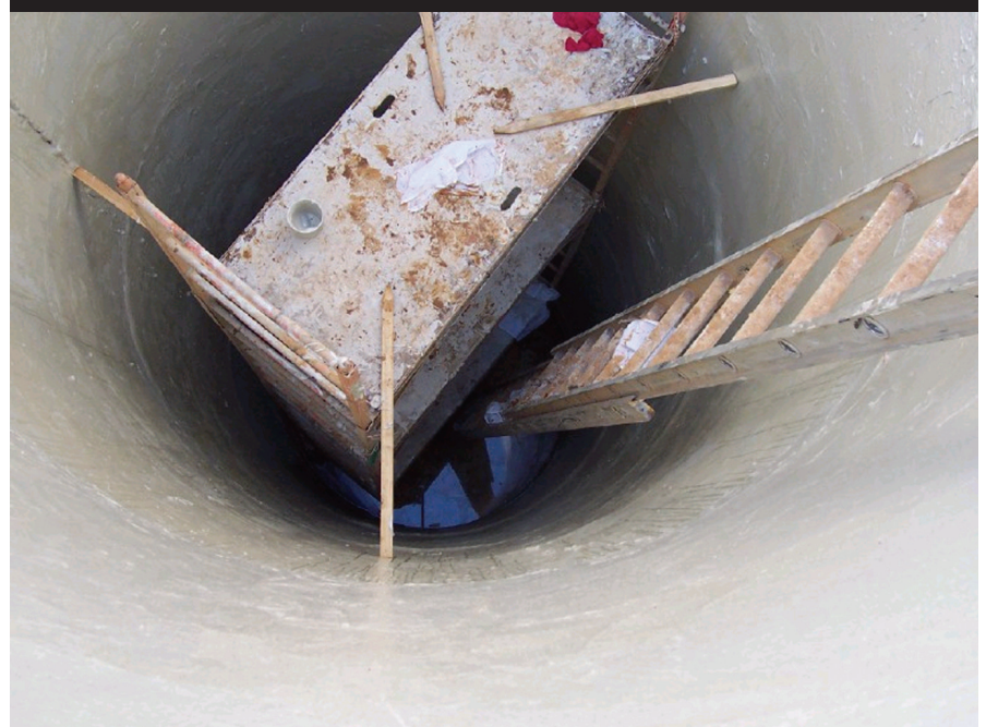
Precast manhole protected from biogenic sulfide corrosion using 100% solids, fiber-reinforced epoxy liner.
