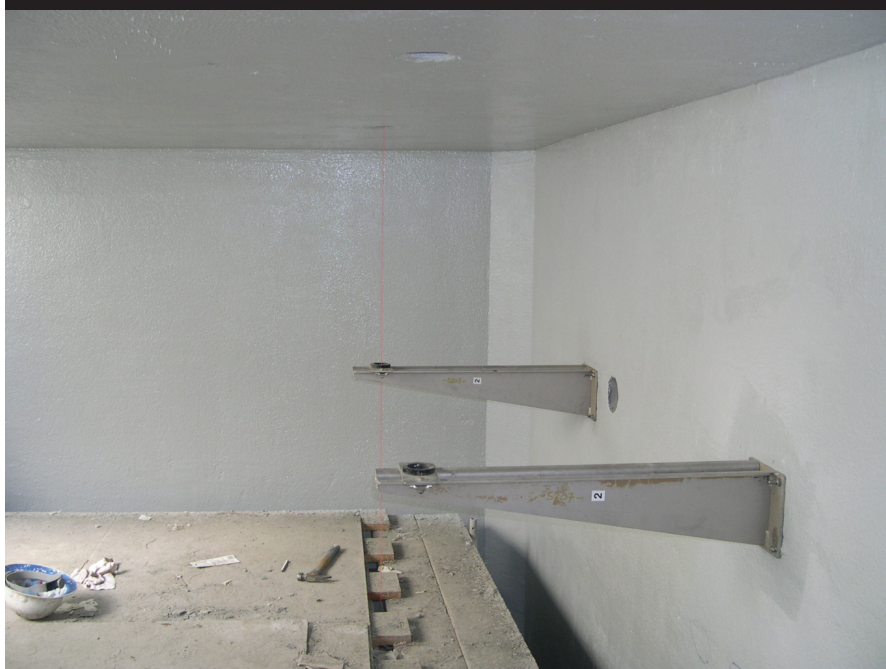
Finished appearance of a lift station restored with an epoxy coating thin overlay, then lined at 125 mils with a 100% solids epoxy mortar and 15 to 20 mils of a 100% solids epoxy glaze coat.
