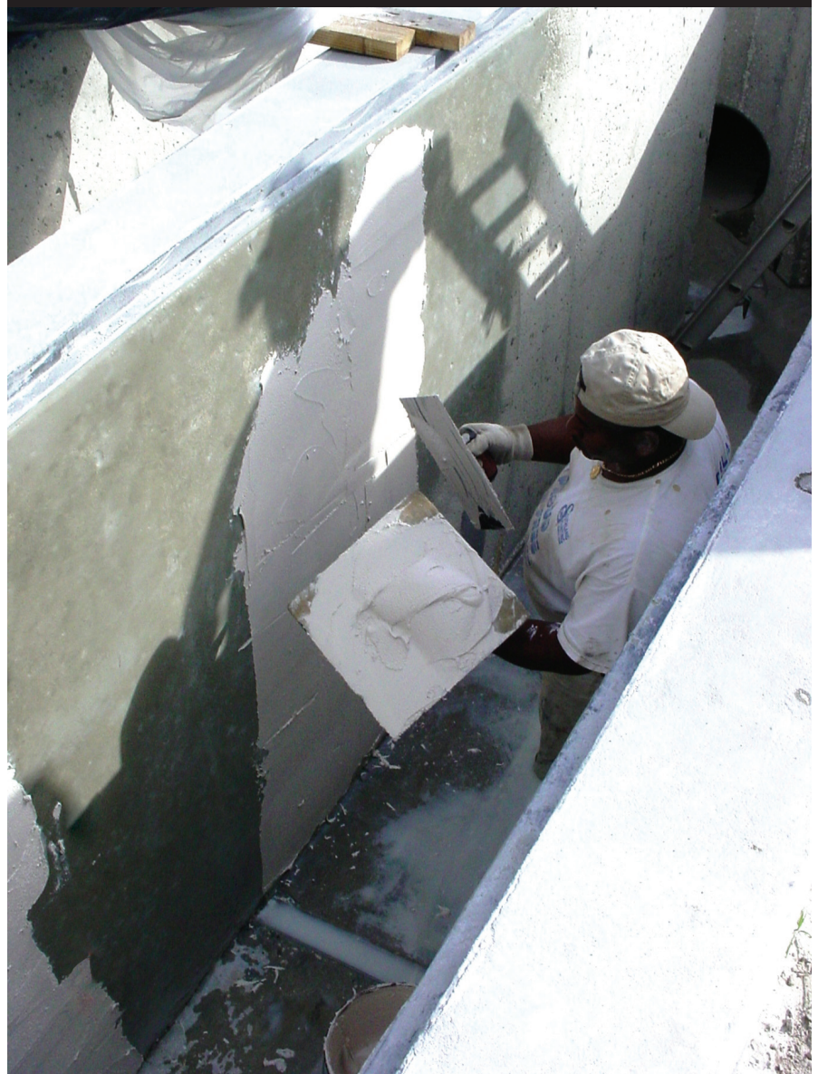
Trowel application at 125 mils of a 100% solids epoxy mortar system designed for elevated H 2 S permeation resistance.
