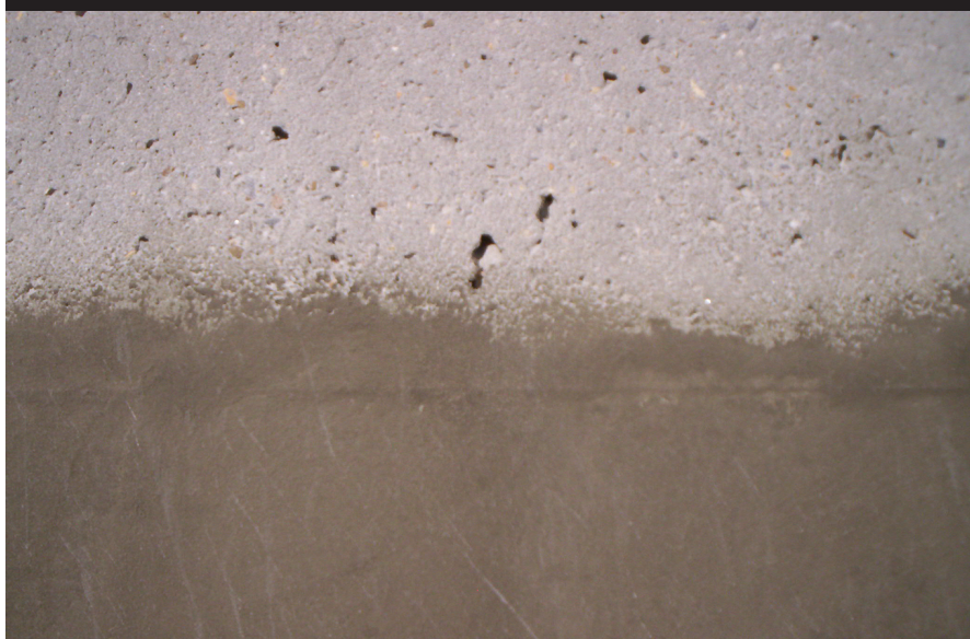
Typical cast-in-place concrete wall containing exposed voids and bugholes (upper half of photo) and application of a greenish-grey epoxy-modified cementitious thin overlay (lower half) to create a contiguous surface for coating.
