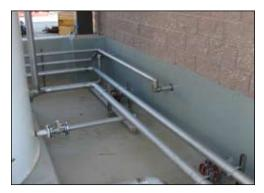
A fiberglass-reinforced coating system from Tnemec protects the secondary containment areas at the Salisbury WWTP from harsh chemicals, thermal cycling, impact and abrasion.
