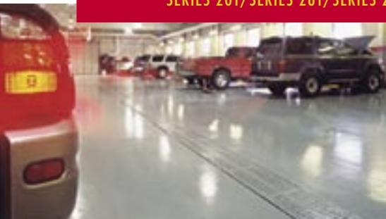
The mechanic's work area of Lewis Toyota is often visible to customers. To maintain its showroom appearance in spite of dropped tools, spilled petroleum products and high exhaust temperatures, an enduring StrataShield flooring system was specified.
