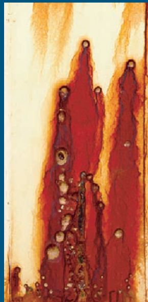
Standard three coats of two-component epoxy
