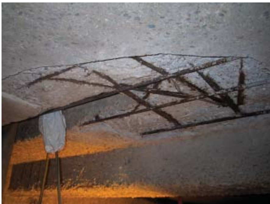
Concrete surfaces after water jetting and hand chipping.
