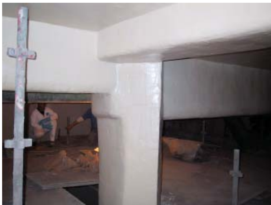
Appearance of the finished coating.
