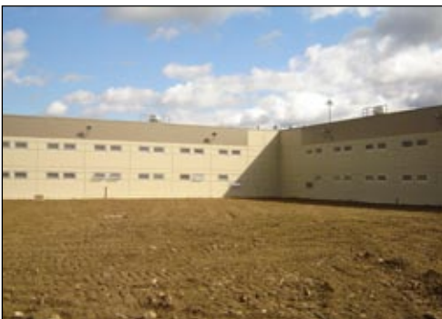
Tnemec coatings were used on both the interior and exterior of the North Branch Correctional Institution in Cumberland, MD.
