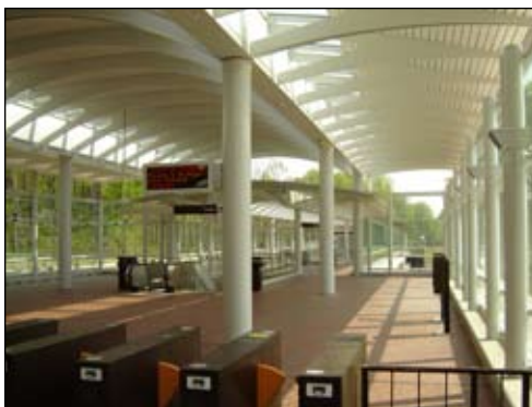
The Largo (top photo) and Morgan (bottom photo) light rail subway stations in Landover, MD are protected with urethane and fluoropolymer topcoats from Tnemec's line of Premier Finishes.
